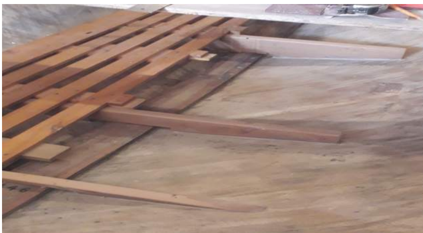
New floors and bottom boards
