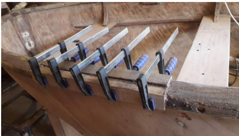
Gunwale and inwhale pieces glued in place
