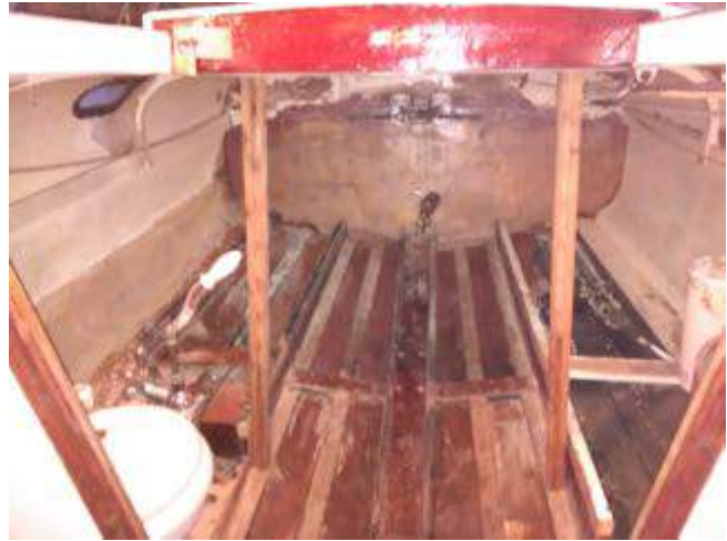
1 Hardwood posts inserted
