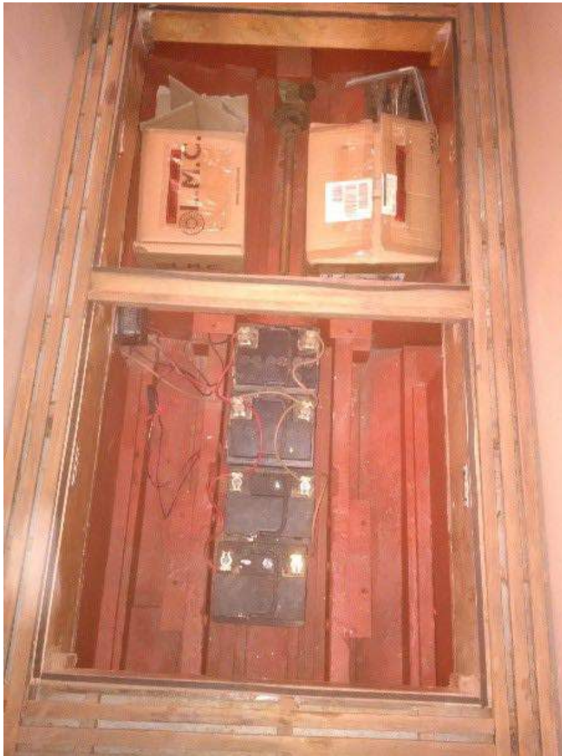
Hatch covers removed
