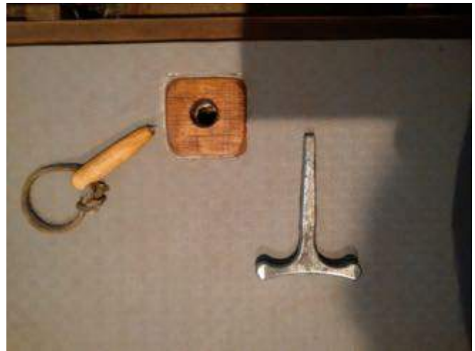
Wood plug and key detail
