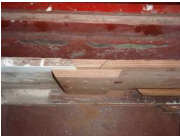
The joint assembled dry. Note the clamp has been removed for this picture to be taken
