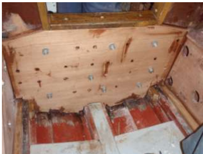
The Forward bulkhead doubler in place. Note the locating blocks at the bottom corners.
