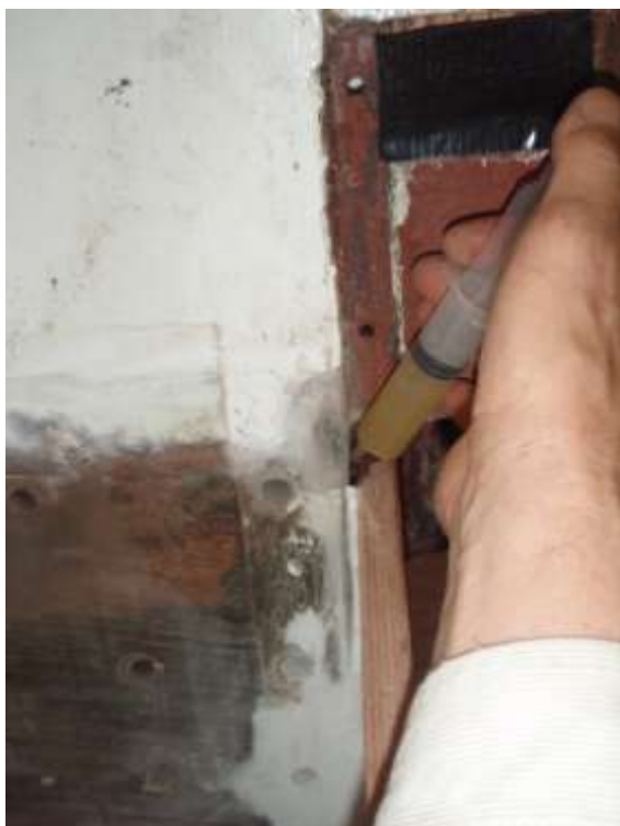
Filling voids with resin.
