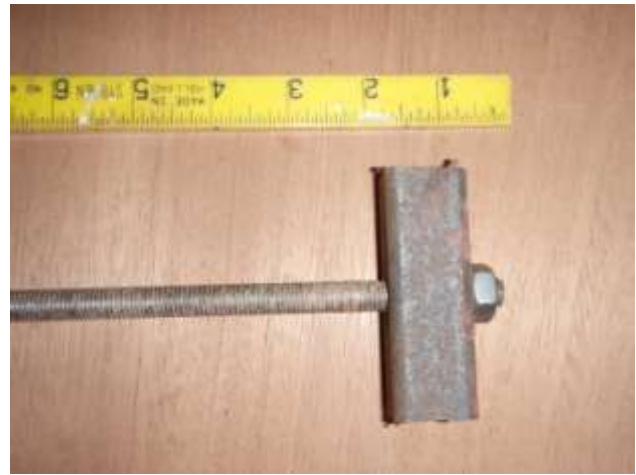
The mechanism for loosening the keel mounting brackets.
