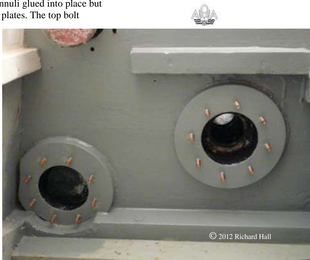
Fig 6: Captive bolts for the bolt access covers
