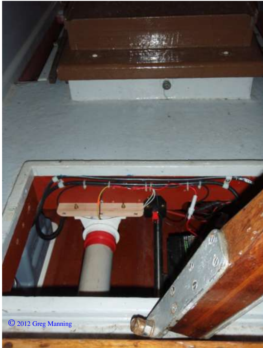
Ducting in place
