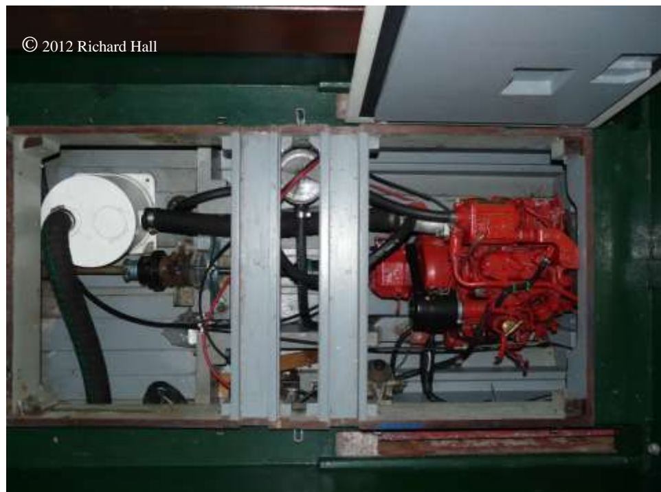
Fig 1: The new engine installation
