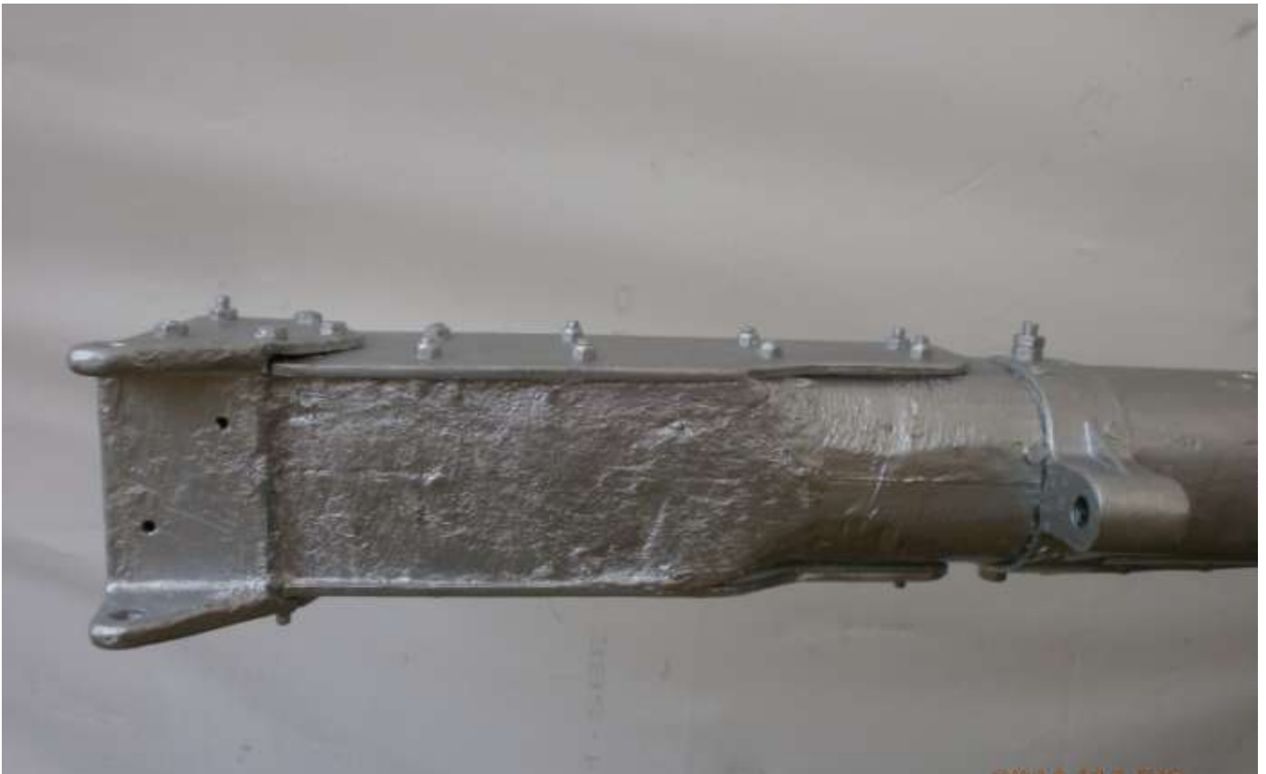
The mast repaired and reinforced
