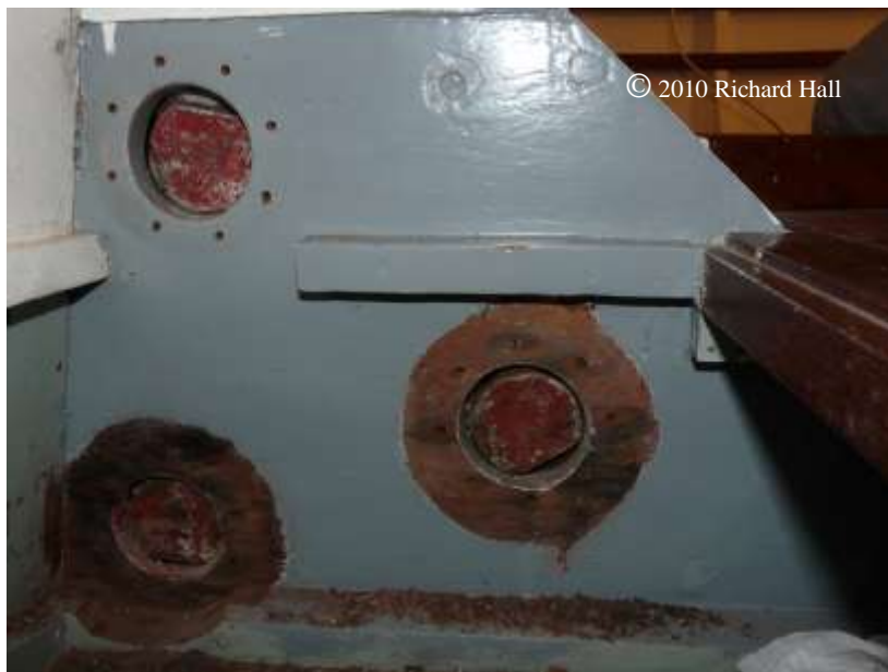
Access holes with cover plates removed
