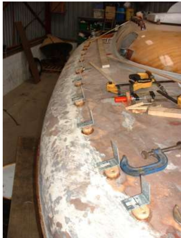
Metal plates in place ready
