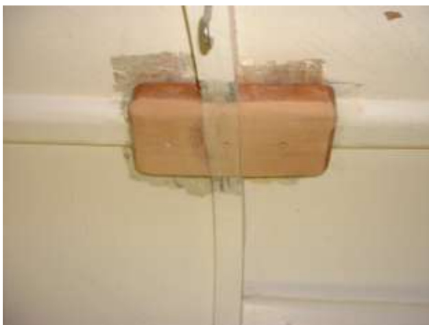
New backing pad in place
