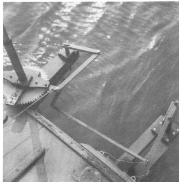
Fig. 2 Tomboy. The rod linkage system.
