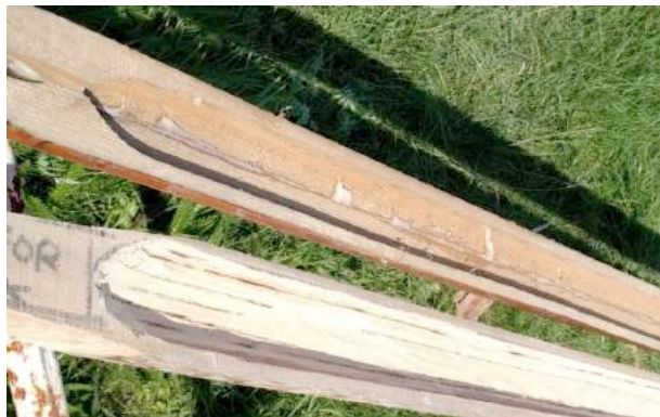
Figure 1. New section routed – taper shaped for gooseneck fitting.
