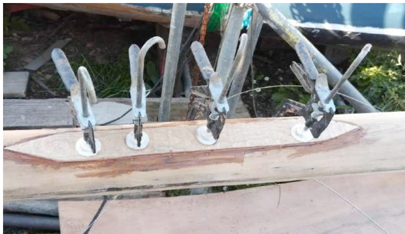
Figure 20. Scarfed graving piece.
