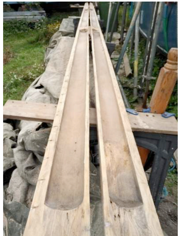
Figure 14 Mast sections after prep clean for repairs.
