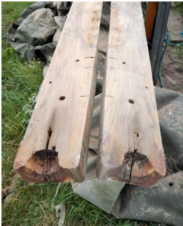
Figure 13. Mast base section – internal view.
