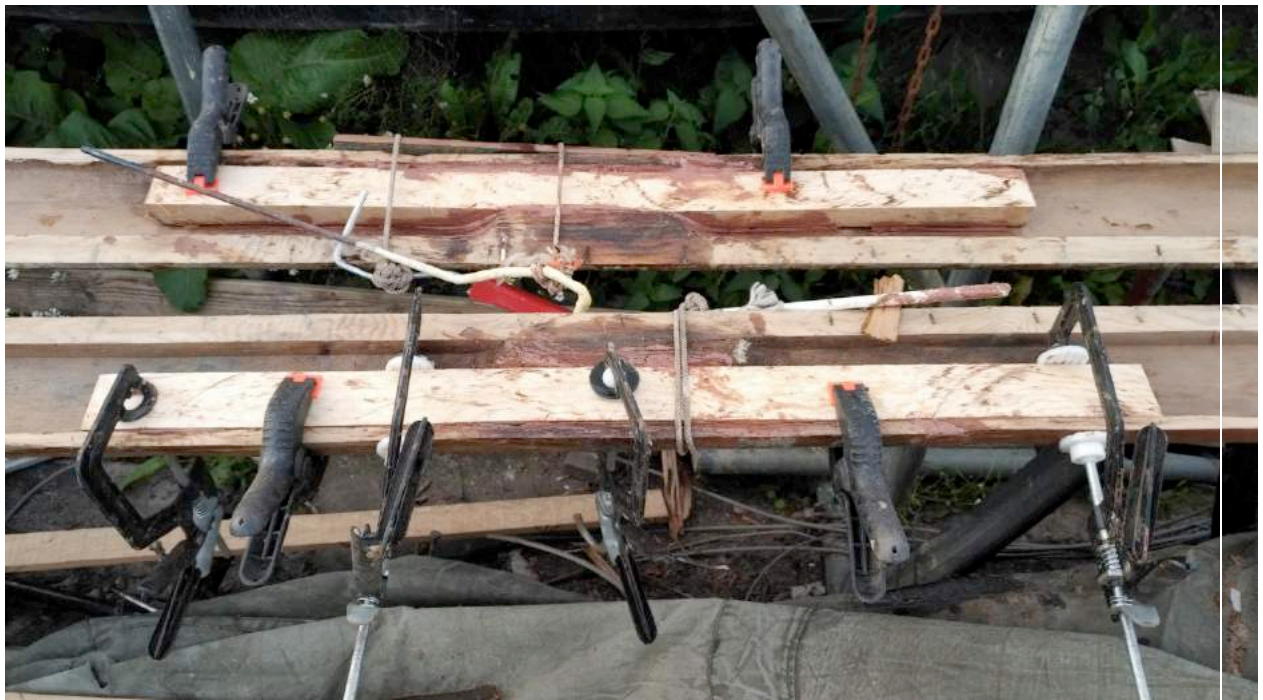
Figure 16. Another view of spruce splines epoxy glued inside crossbeams.
