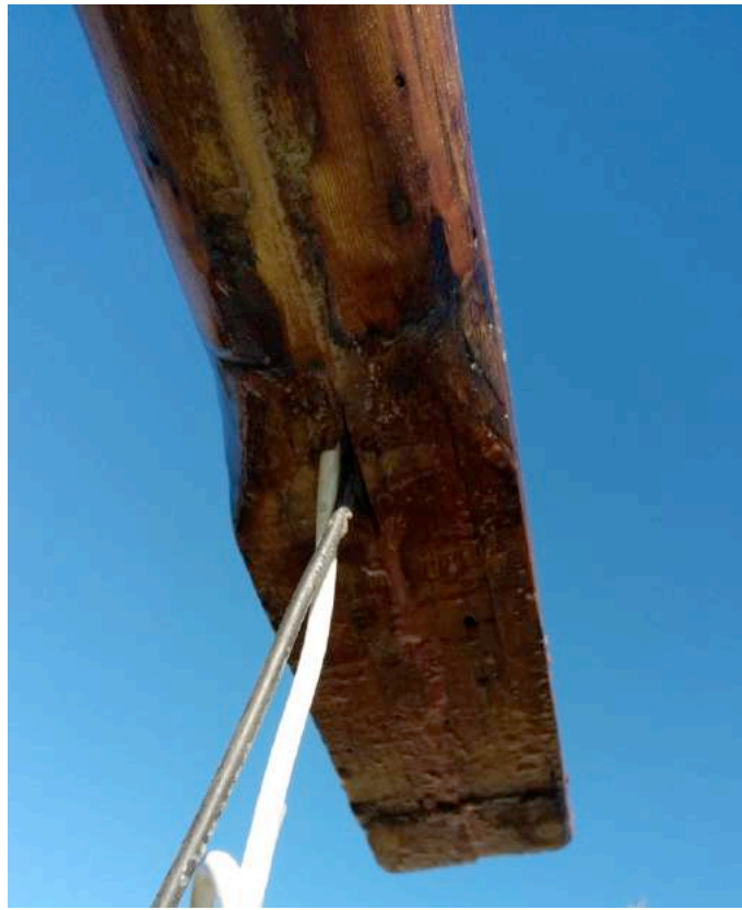
Figure 23. Cable routing at mast base.
