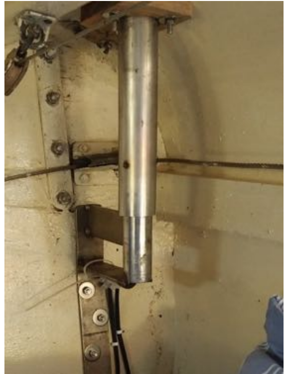
Supporting the base of the mast
