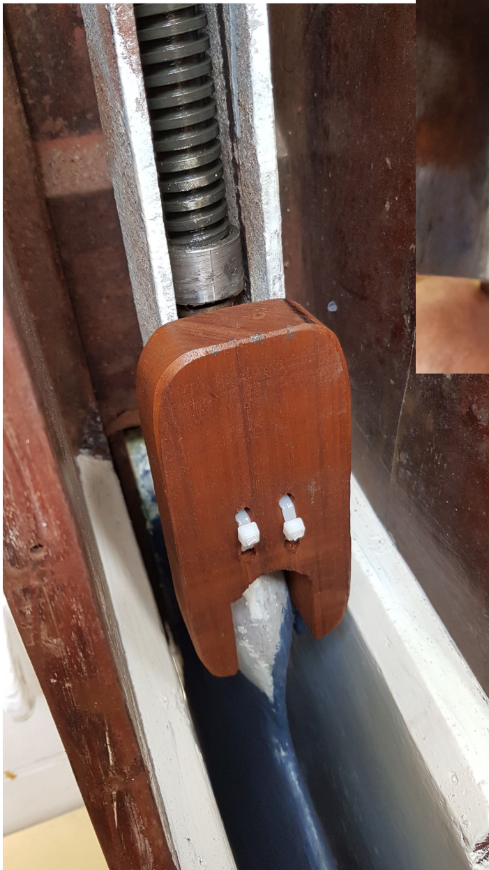
Block cable tied in place
